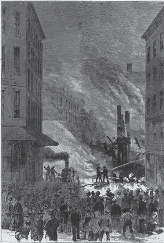
THE BOSTON FIRE—WASHINGTON STREET, LOOKING NORTH, WITH RUINS OF THE CHECKING BUILDING AND GRAND THEATRE ON THE LEFT.
