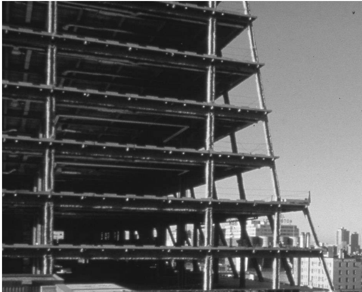
Figure 9 : vue d'une structure mixte, Thrivent Financial Building, Photo de City of Minneapolis Archives
